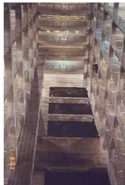
Providing a light well at the center of a parking structure can bring daylight into the center of a wider building, minimizing lighting needs during the day, as in this example at Wells Fargo Financial in Des Moines, Iowa. Engineer: Walker Parking Consultants
